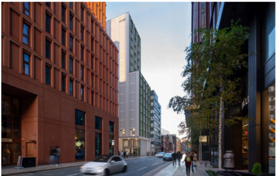
VIEW FROM CHARLES STREET (WEST)
