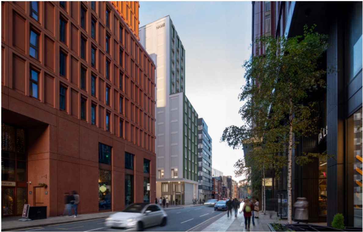
VIEW FROM CHARLES STREET (WEST)
